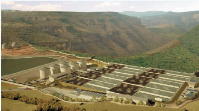
Image of Agua Prieta wastewater treatment plant in the State of Jalisco. Source: Mitsui & Co., Ltd.
