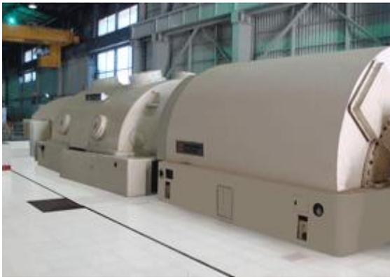
Geothermal Steam Turbine Generator previously delivered to Cerro Prieto power station in Mexico
