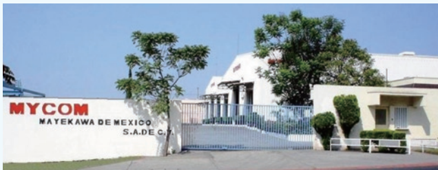
Mayekawa's plant in Morelos, Mexico
